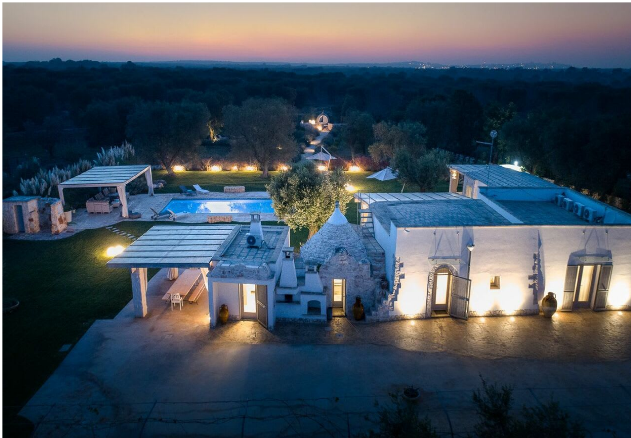
Aerial view of the property at night
